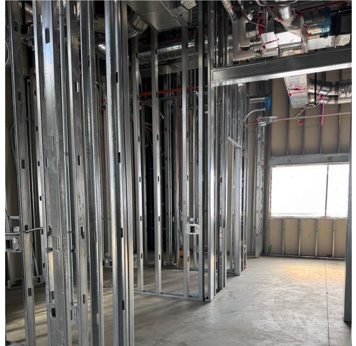
Terminal Interior Framing
