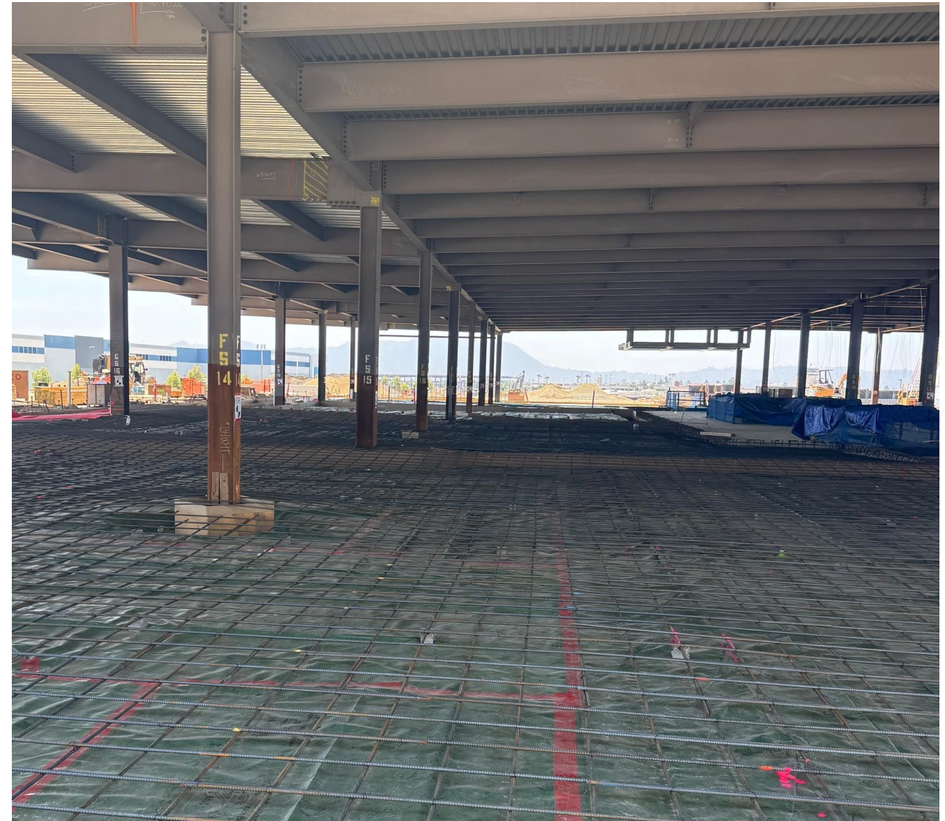
Terminal Area D Steel and Slab Rebar
