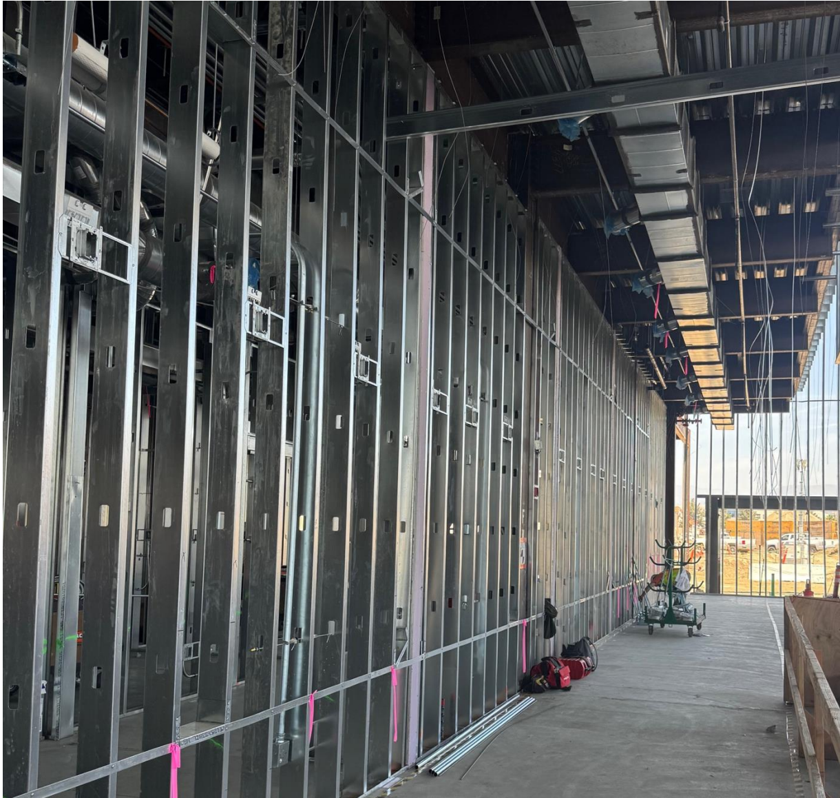
Terminal Check-In Framing
