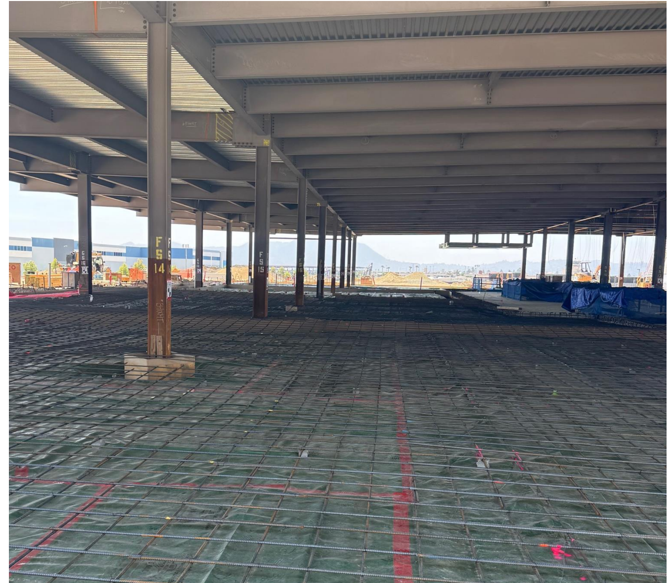
Terminal Area D Steel and Slab Rebar
