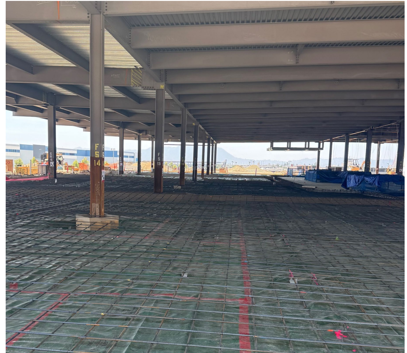
Terminal Area D Steel and Slab Rebar
