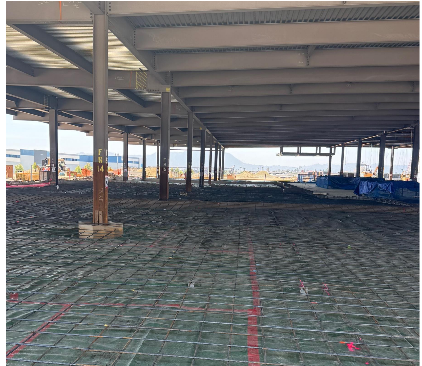
Terminal Area D Steel and Slab Rebar
