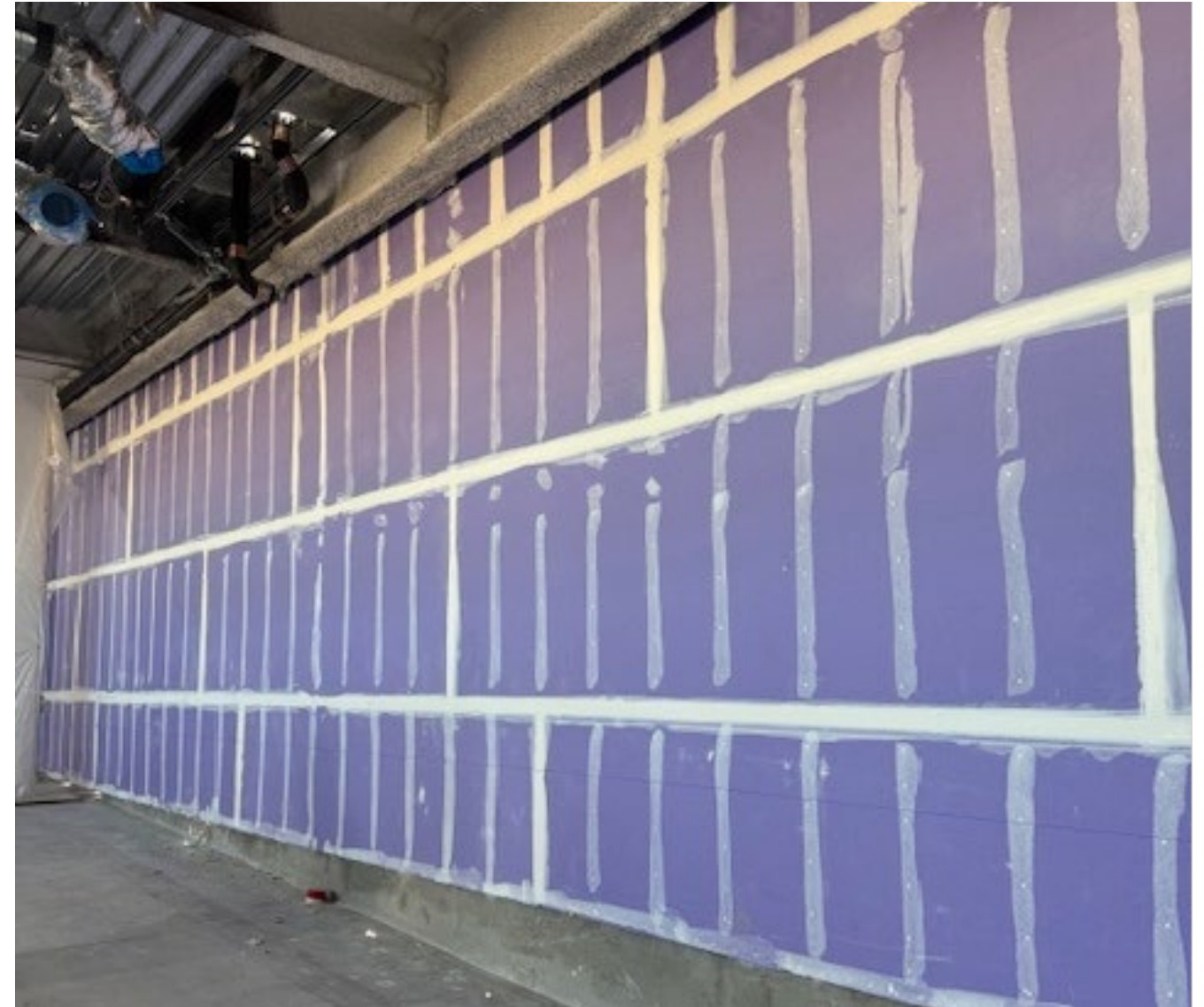
Concourse Connector Drywall
