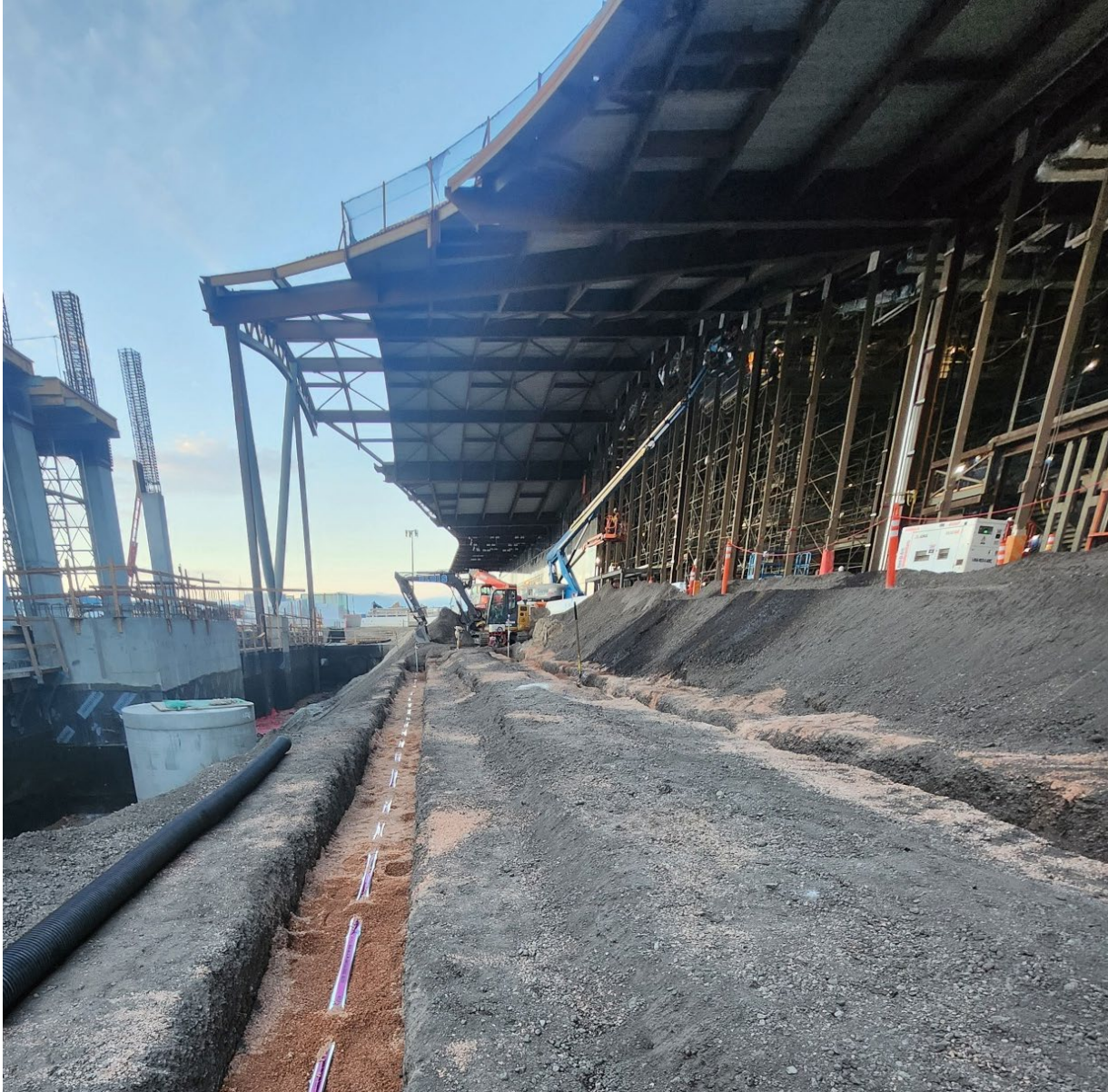
Underground Utility Installation
