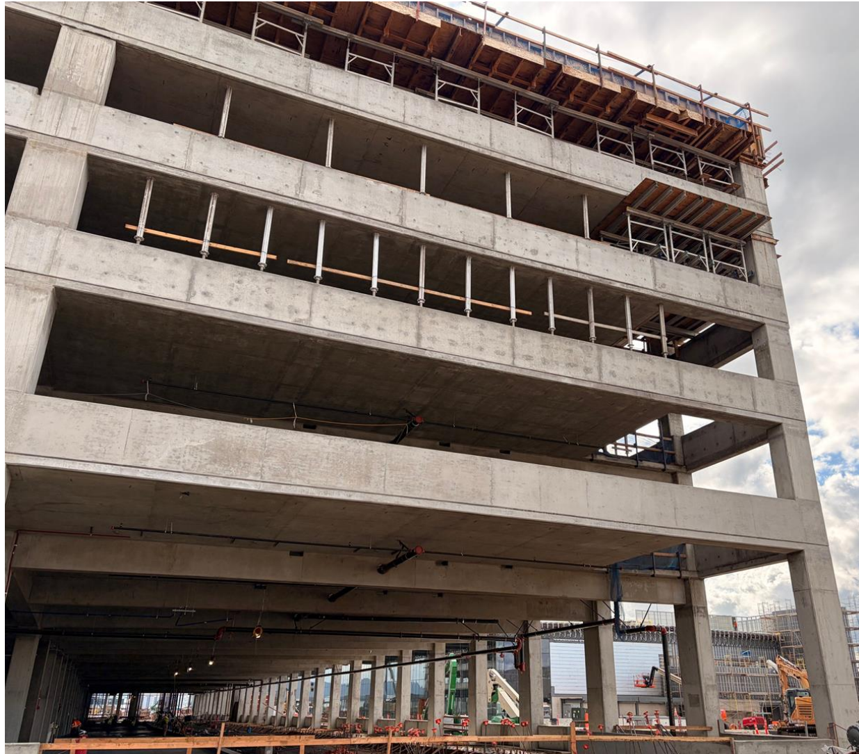
Parking Garage Exterior
