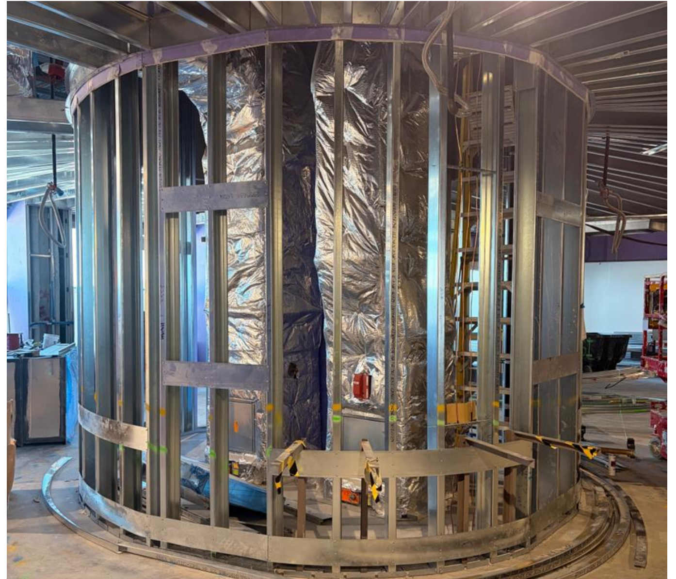
Terminal Level 2 Curved Framing
