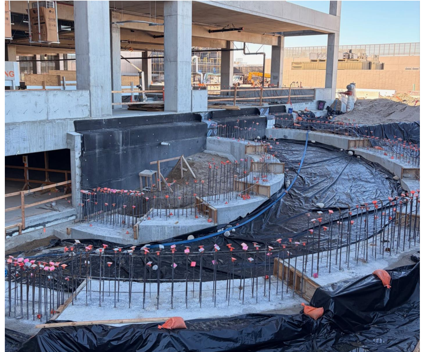
Garage Helix Ramp Foundations
