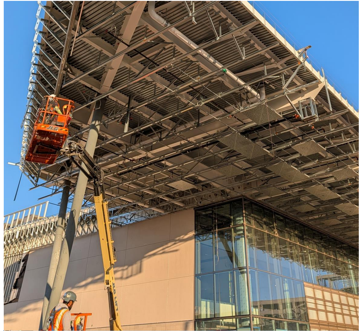
Area C Fascia/Soffit Framing
