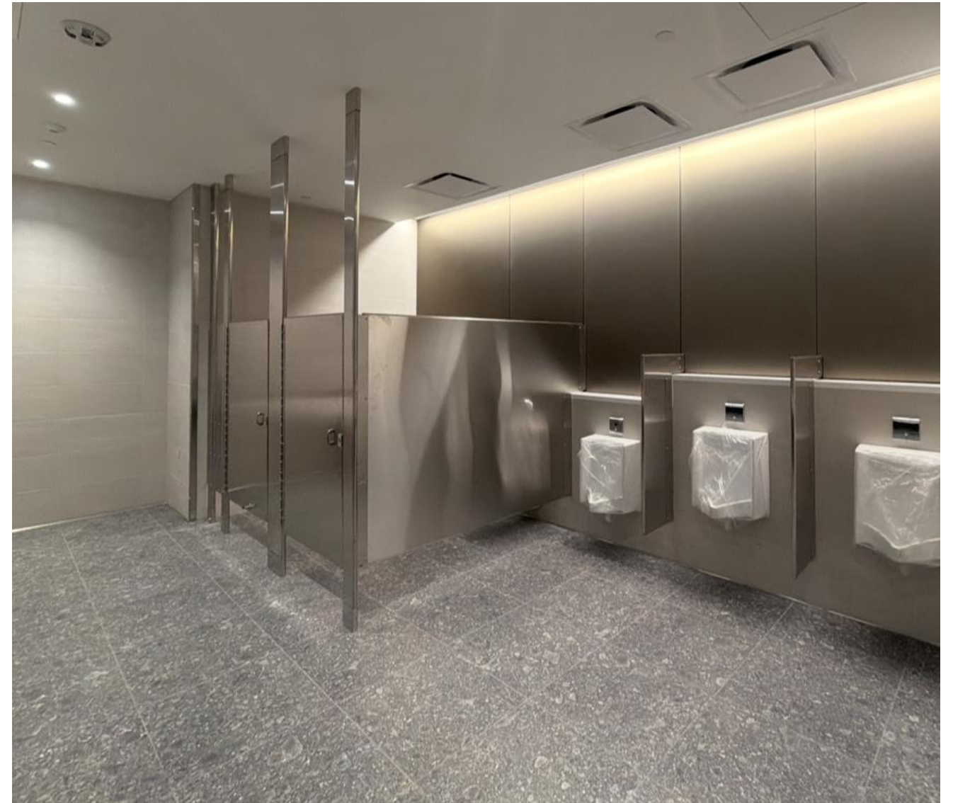
Completed A Restroom
