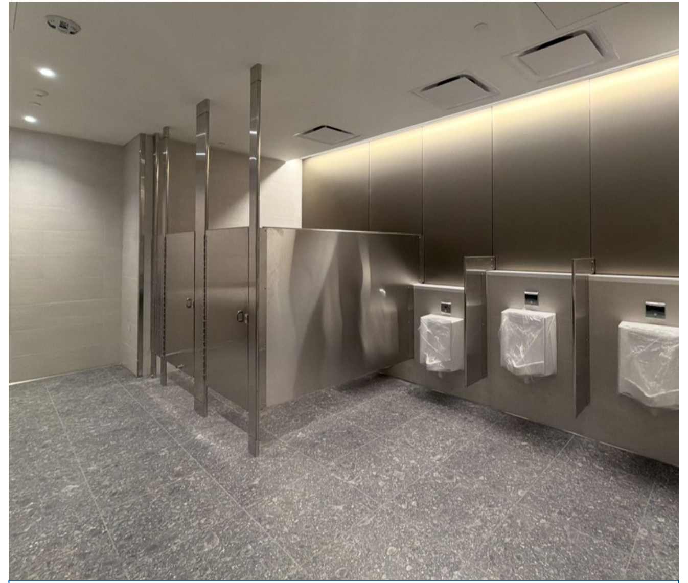
Completed A Restroom
