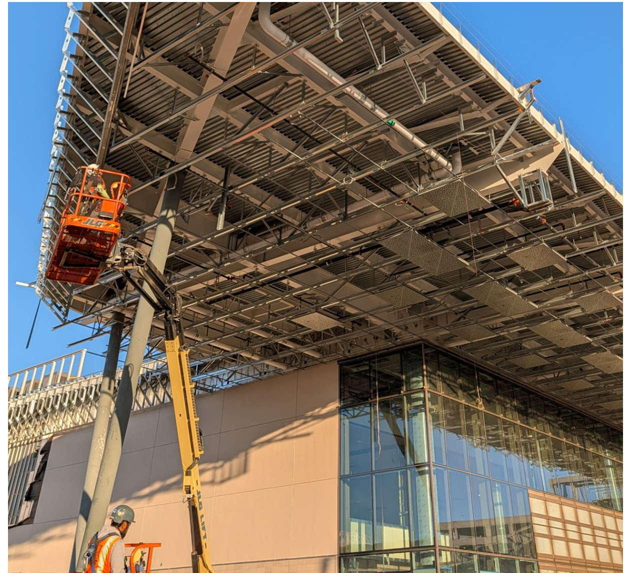
Area C Fascia/Soffit Framing
