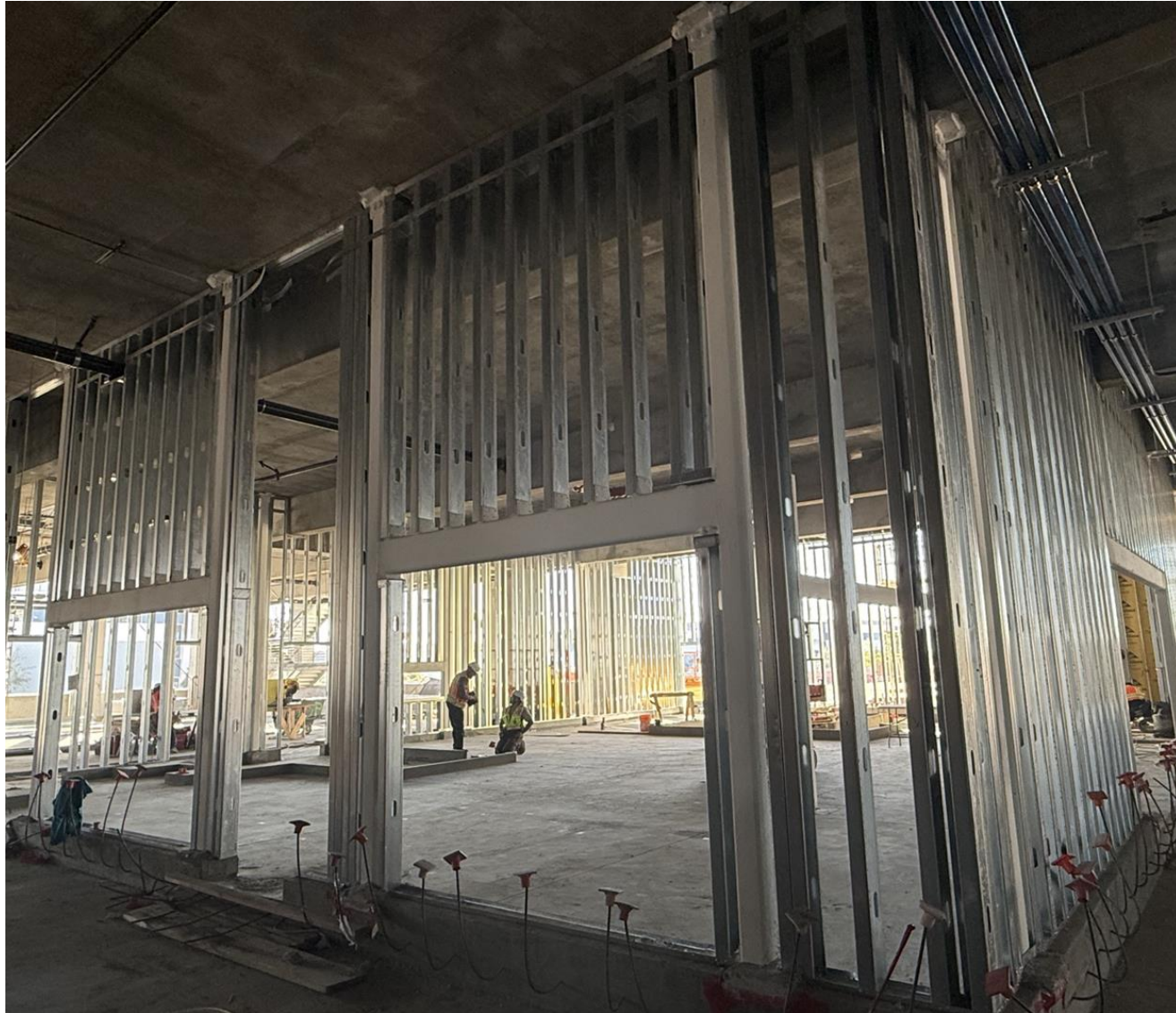
Garage Valet Office Framing
