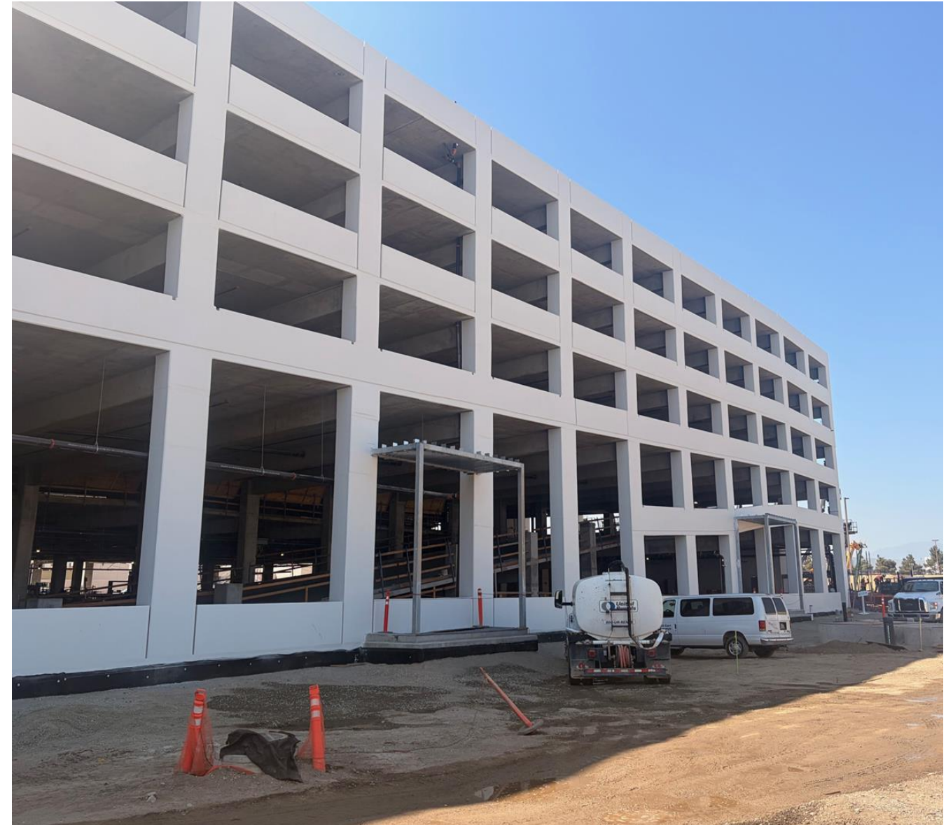
Garage Exterior Coating
