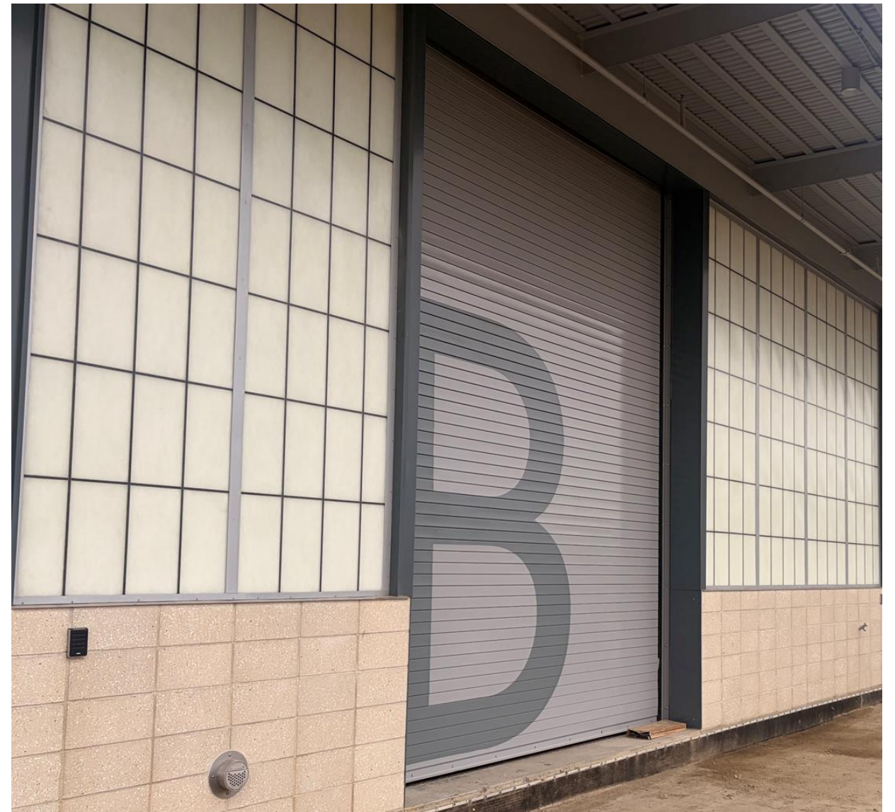
ASF Overhead Door
